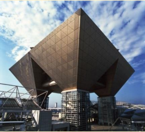
Framed structure (Tokyo Big Sight)
